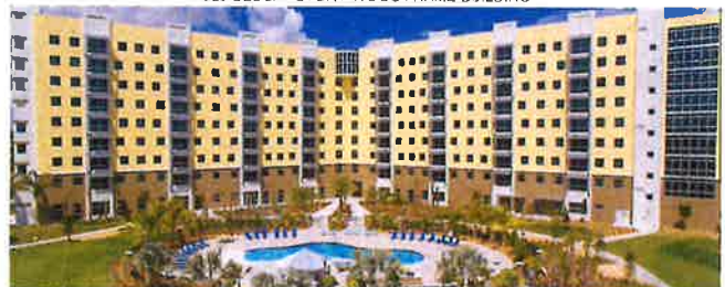
Florida International University, Bayview NORTH MIAMI, FL 410 BEDS/NINE-STORY HIGH RISE BUILDING
